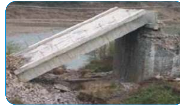
A Bridge in Jhelum Valley, AJK Old ? New ?
