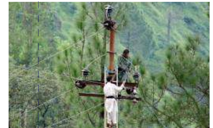
Electricity being restore in EQAAs
