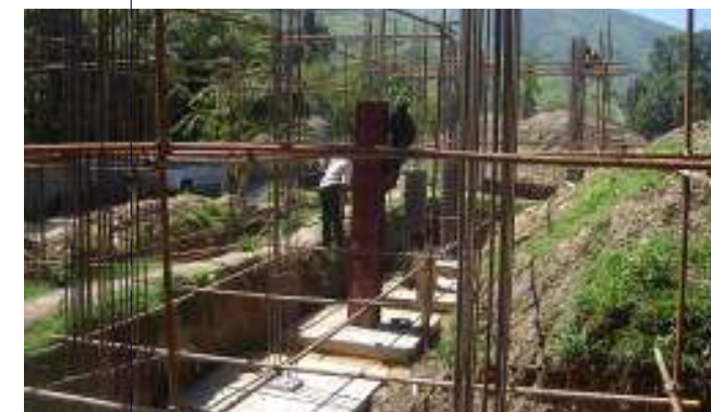
Construction work underway
