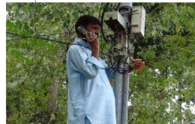
Telecommunication Network being restored
