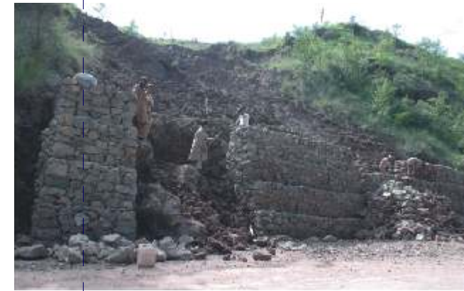
Slope Stabilization in EQAAs
