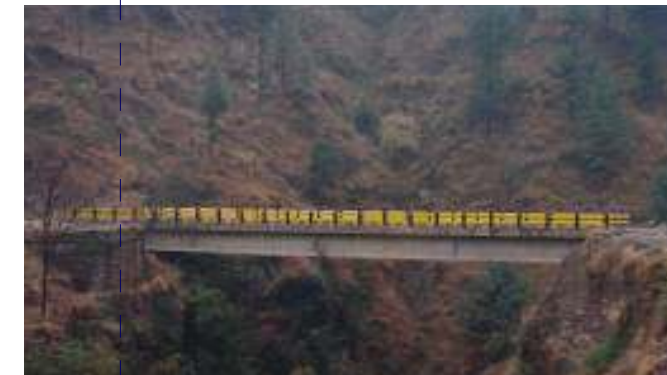
Newly constructed bridge on Jhelum Valley Bridge
