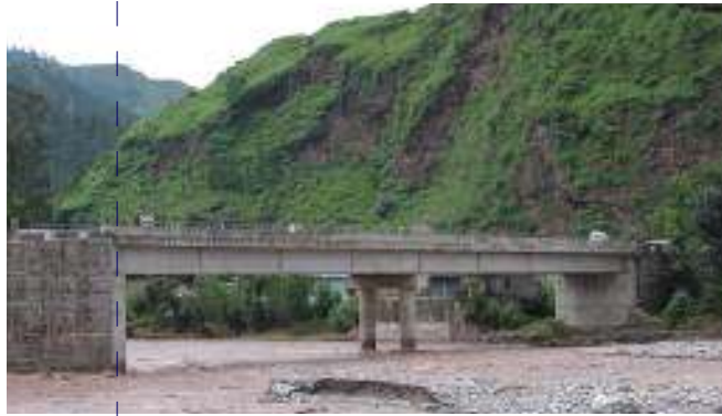
Reconstructed Gari Habibullah Bridge
