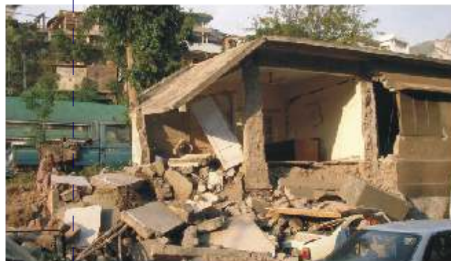
A Destroyed House in EQAAs
