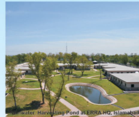
Rainwater Harvesting Pond at ERRA HQ, Islamabad
